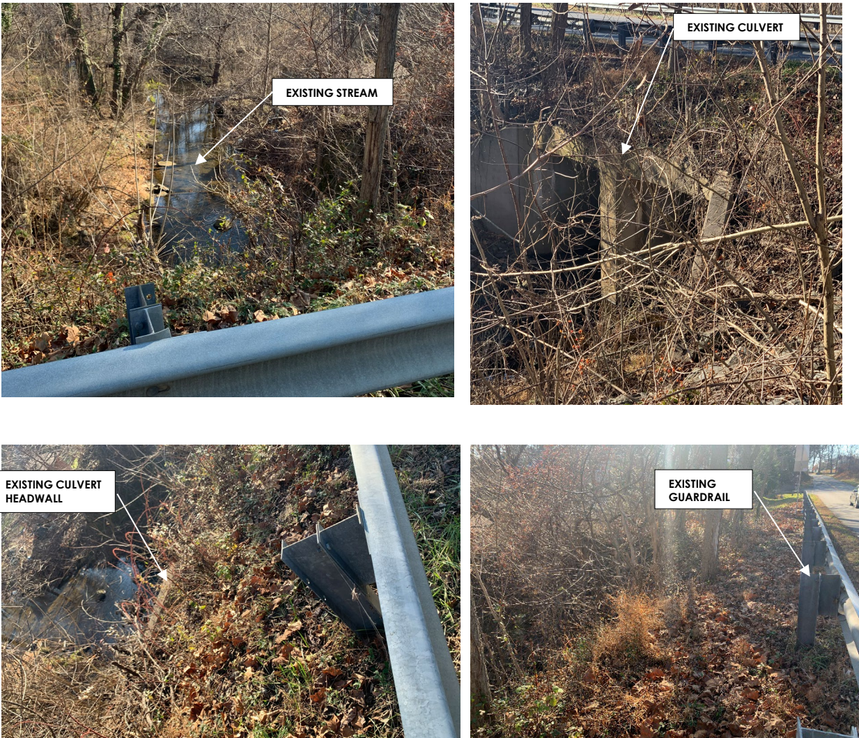
Figure 6 - Existing Box Culvert
