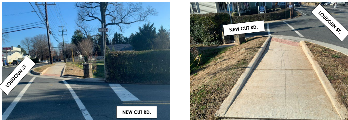
Figure 2 - Existing Ramp at Loudoun St
